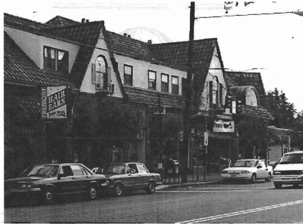
Residential units above commercial streetfront.
