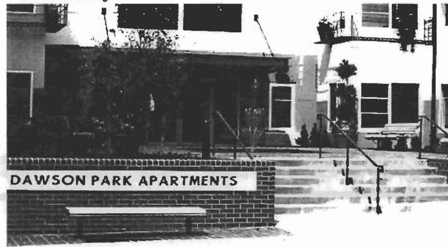
Benches & low walls enhance the streetscape.
