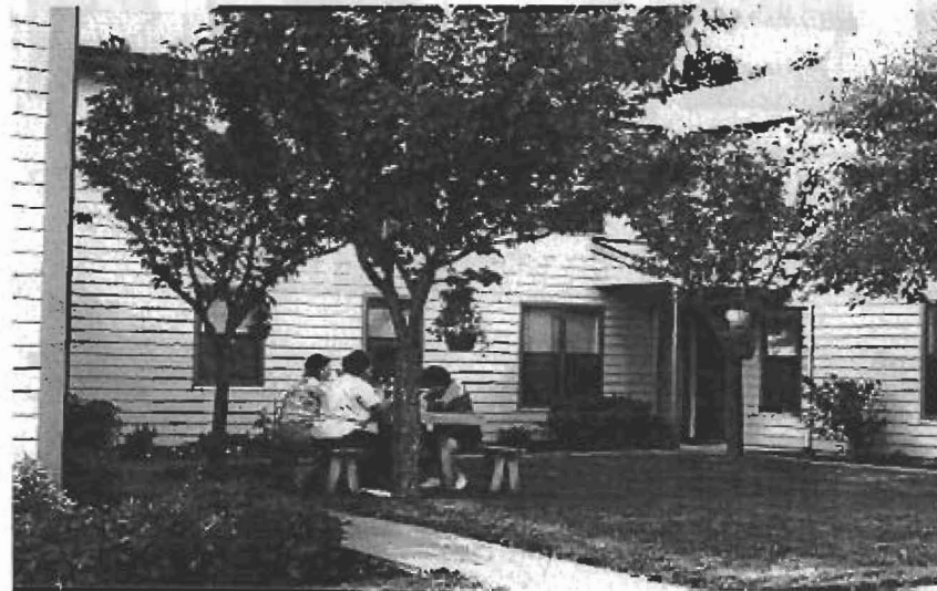
A shared courtyard.
