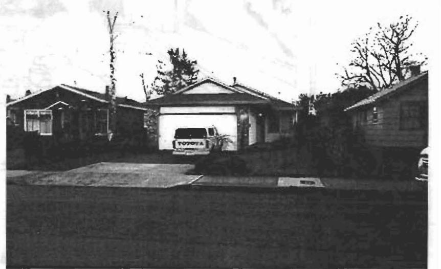
Garage dominates the streetfront / excessive paving.
